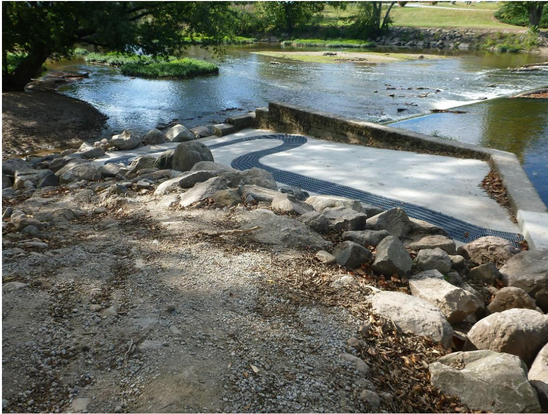
Figure 6. Fish ladder at the Stockdale dam in the Eel River near the town of Roann, Indiana. The fish ladder is a prototype approach to providing fish passage around the dam.
