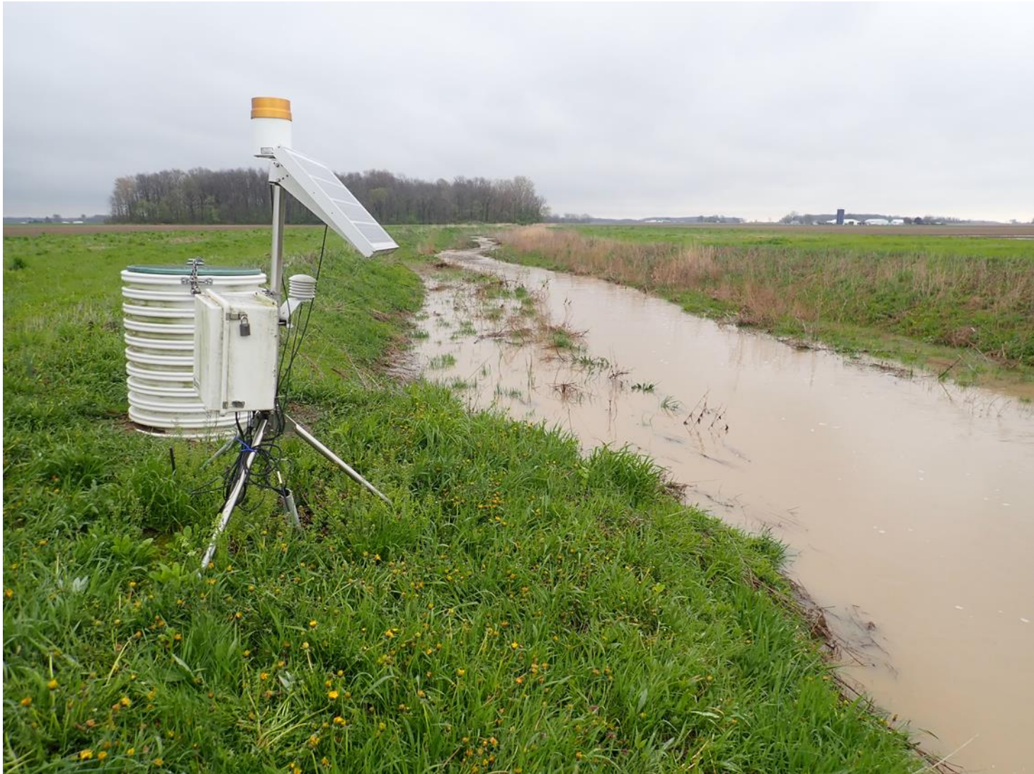
Figure 4. Upper Beargrass Creek natural channel design during flood event. There is a 120-foot prairie grass mix planted as a buffer and to improve wildlife habitat. Bank erosion has been significantly reduced to the previous trapezoidal wooded ditch. This design is the future to improve farm drainage, provide improved fish and wildlife habitat and improve bank stability.
